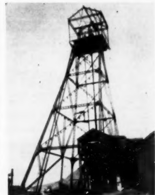
Steel Mine Head Frame
